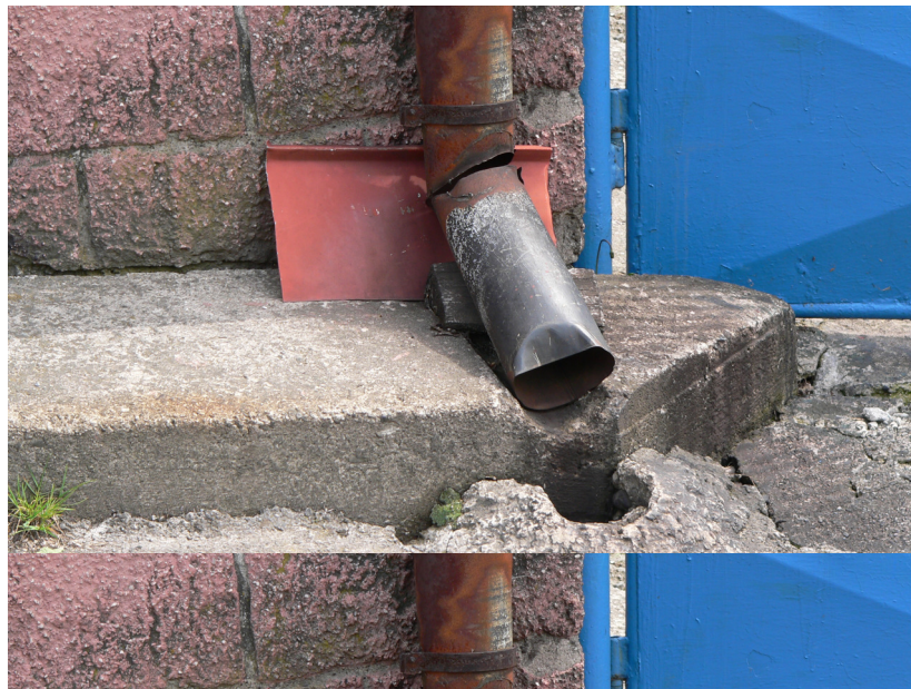
Fig. 13 The sluicing away rainwater
