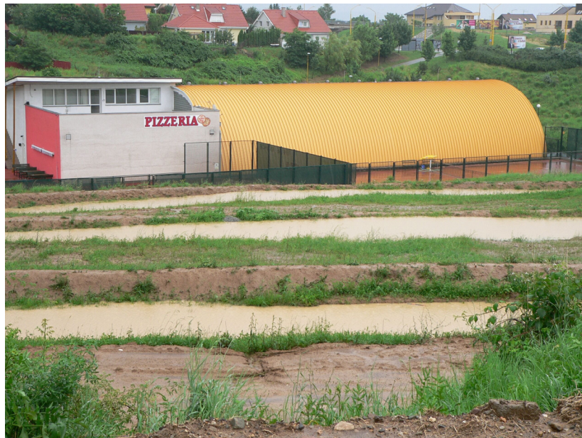
Fig. 36 The KVP housing estate in Košice – protection of buildings under a slope with the help of earthen bunds along contour lines
